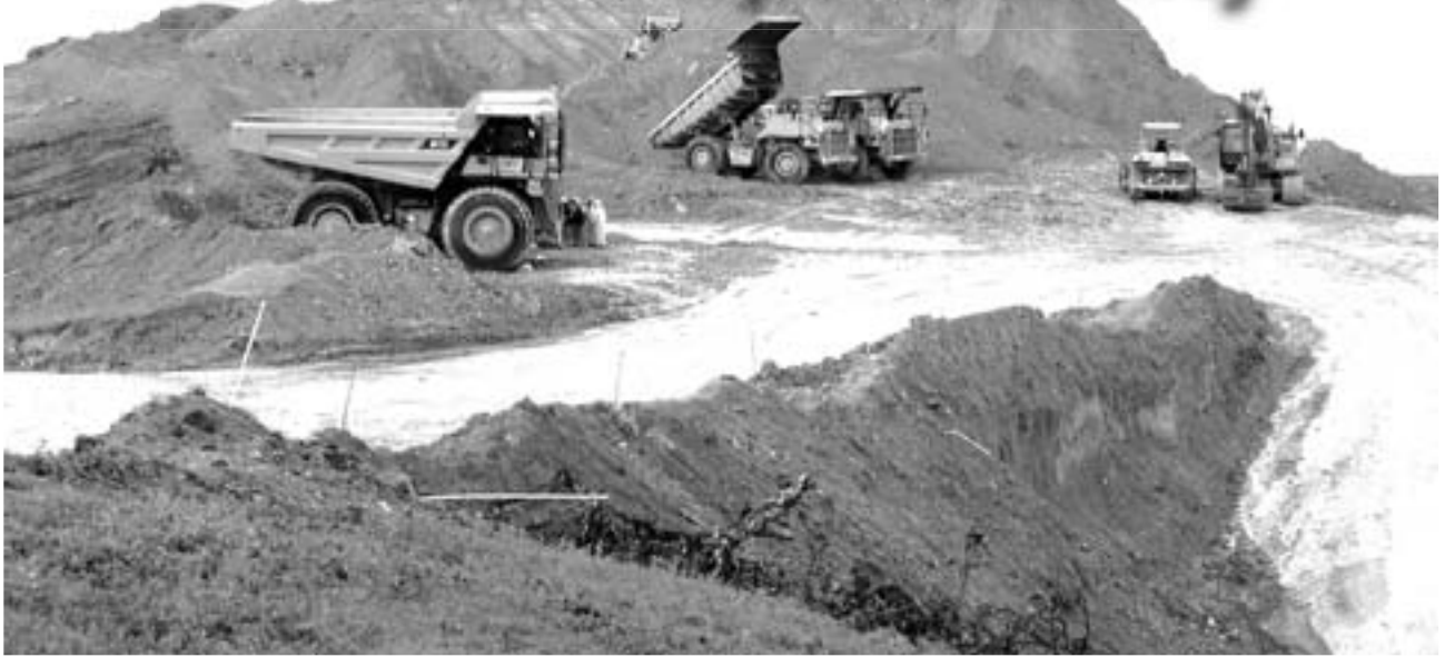
Mining operations in Guatemala
